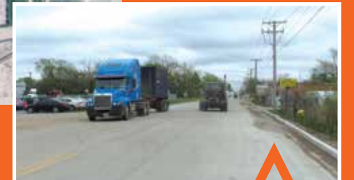
167th Street (CN Terminal/Harvey and South Holland Industrial Districts): Under Construction
