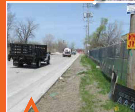
Center Street (CN Terminal/Harvey Industrial District): Under Construction
