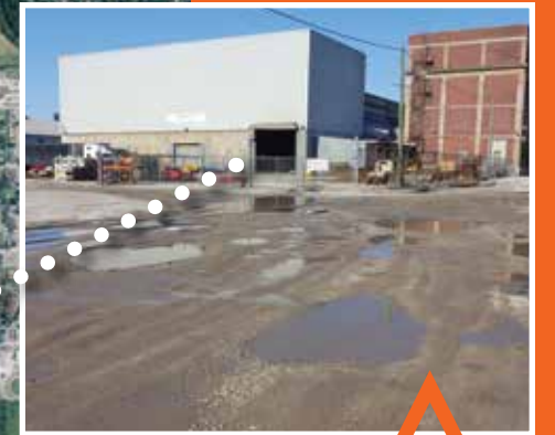
156th Street (LB Steel): Under Design
