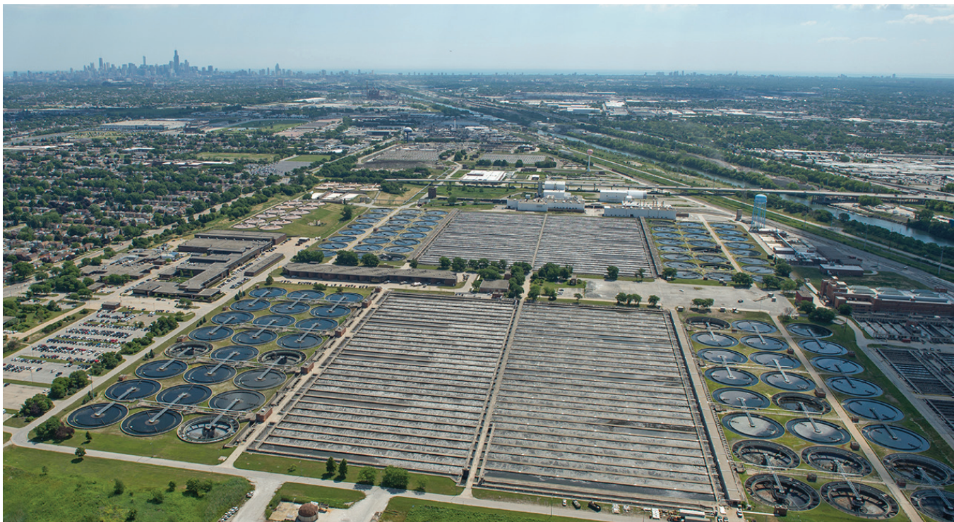
Stickney Water Reclamation Plant
