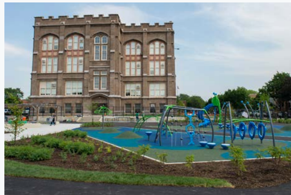
Davis School before (L) and after (R).
